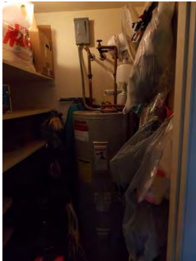
Each apartment has its own electric-heated DHW tank.
