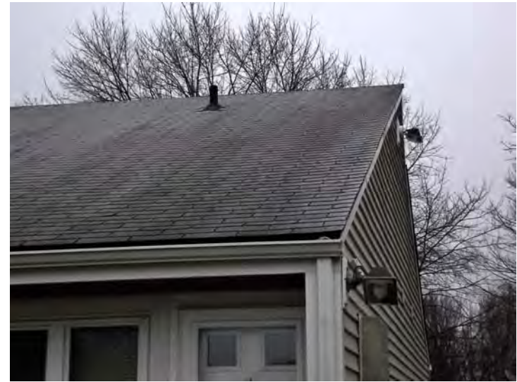
Roofs are covered with asphalt shingles, and each building has gutters and downspouts.
