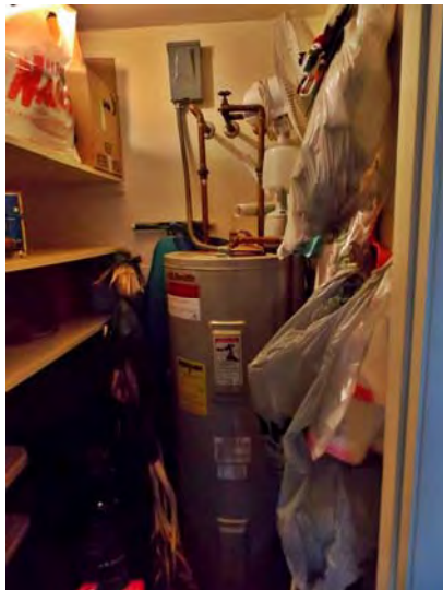
This is one of the electric-heated DHW tanks.
