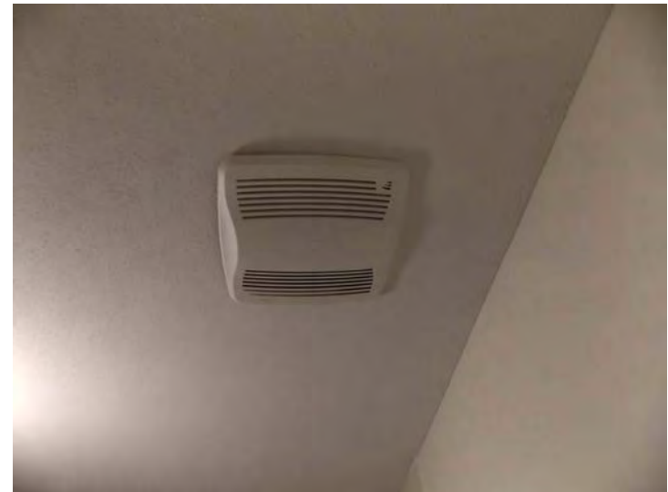
Bathrooms have also been recently upgraded with exhaust fans that respond to humidity levels.
