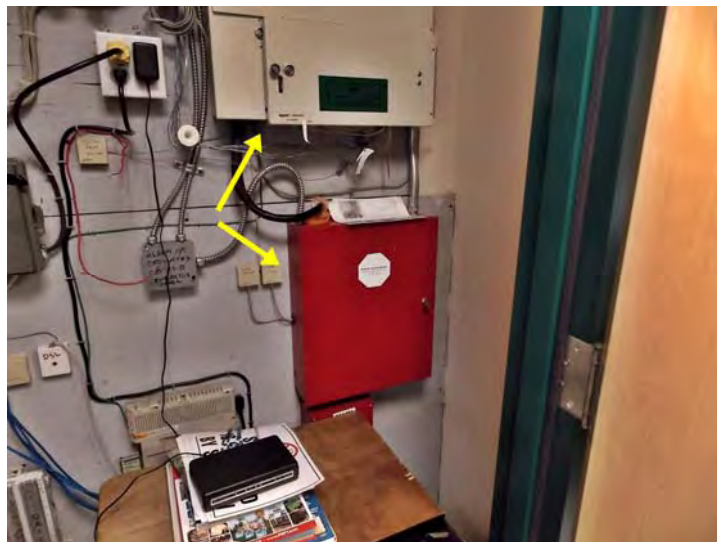
The central fire alarm control panel (FACP) is located in the community building (at the adjacent Snipsic Village I).
