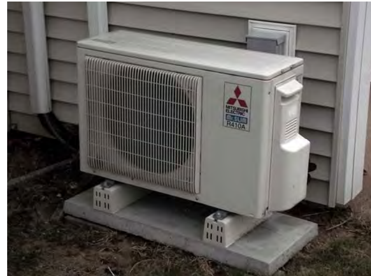
Each unit has an air-cooled pad-mounted heat pump condenser.
